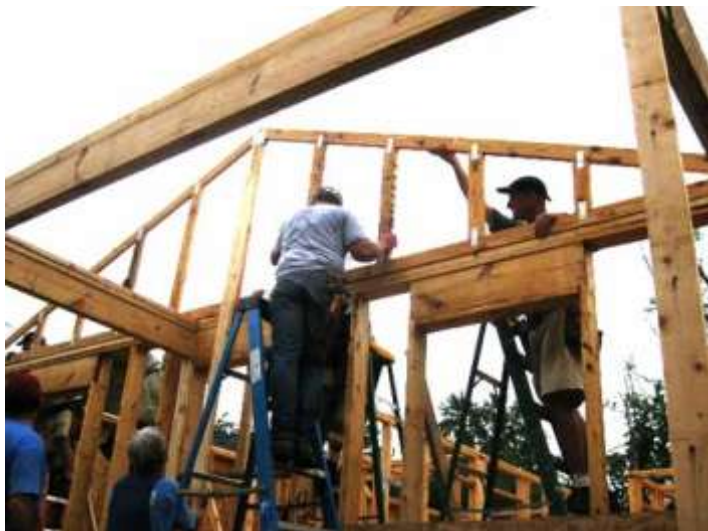
St. Mark's Habitat for Humanity work crew
